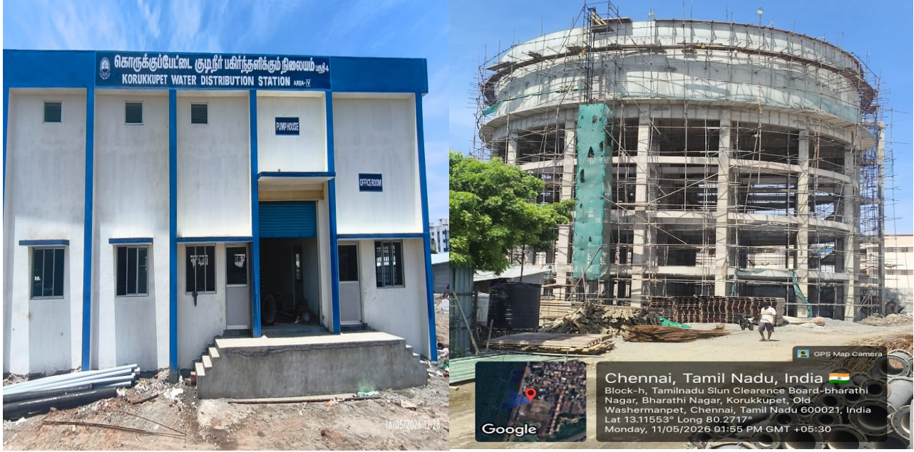
construction of 10 MLD Underground Reservoir, 3 MLD Overhead Tank & 600 mm DI Transmission Pipeline Location: Bharathi Nagar, Korukkupet, Chennai, Tamil Nadu
