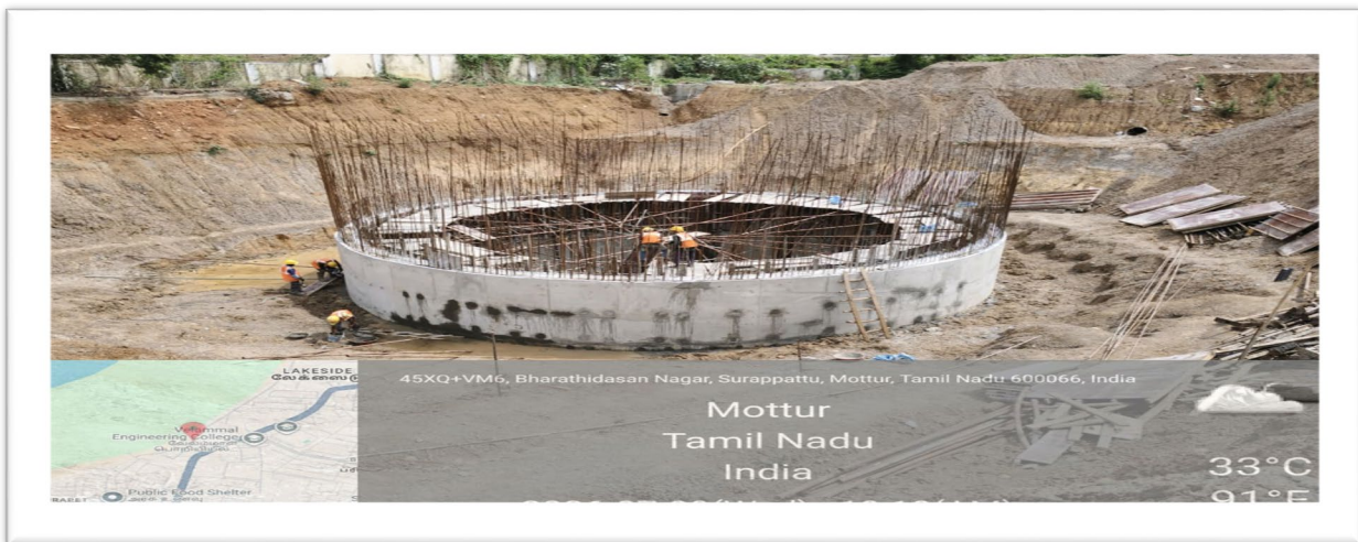
Design, Build, Operate & Transfer of 47 MLD Water Treatment Plant (WTP) Including Comprehensive Operation & Maintenance for 10 Years Location: (📍) Surapet, Chennai
